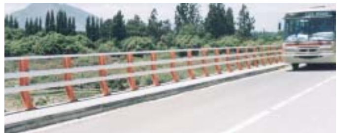
Maipo River Bridge, Naltagua Valley, Chile
